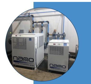
hot, moist compressed air enters the separate air to air heat exchanger where it is precooled
